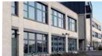
Leister Technologies GmbH, Aachen, Germany
