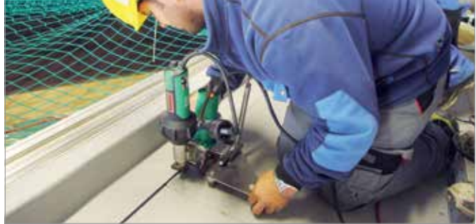
Greater stability and reliability in device guidance thanks to the welding guide.
