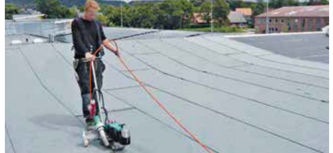
Easy unit guidance and clean working with the BITUMAT B2.
