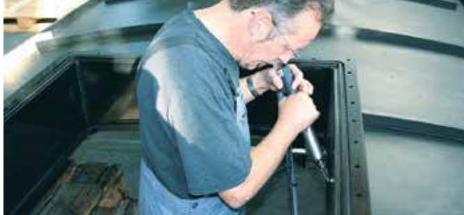
Draw welding on a PE-container with the DIODE PID.
