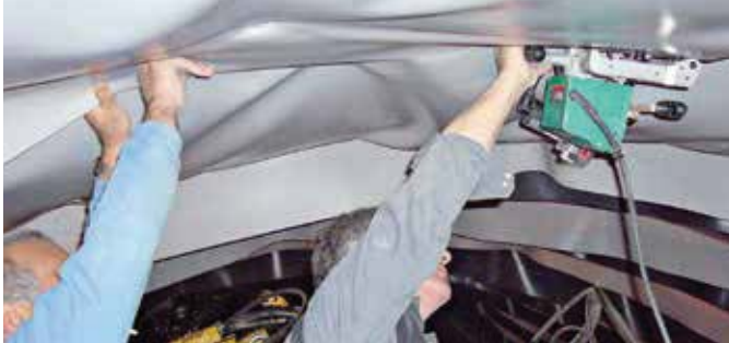
Comet operating in the tunnel ...
