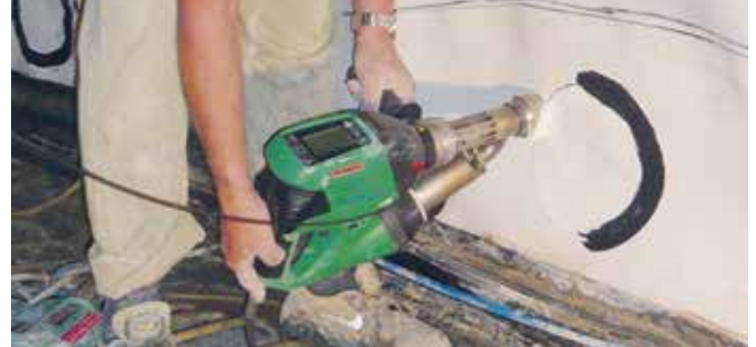
The robust WELDPLAST S2 welding a patch in a tunneling application.
