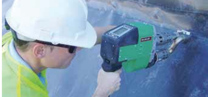
The powerful WELDPLAST S4 at work.
