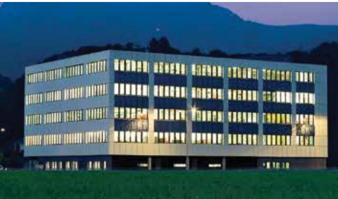
Leister Technologies AG, factory, Samen, Switzerland
