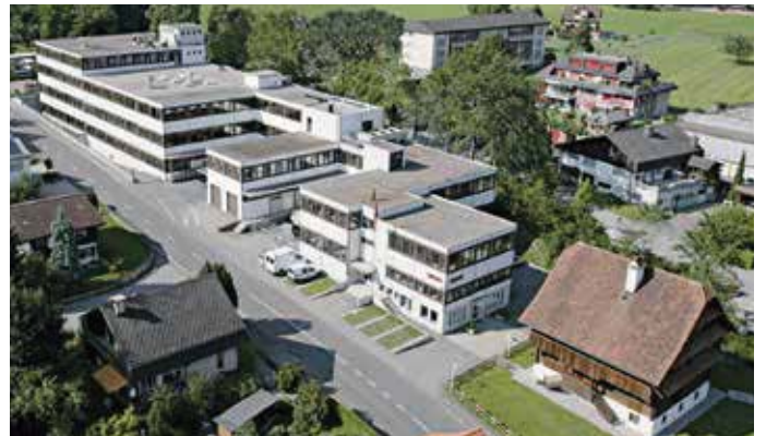
Leister Technologies AG, factory, Kaegiswil, Switzerland
