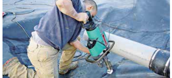
WELDPLAST S6 undertaking assembly applications on a landfill site.
